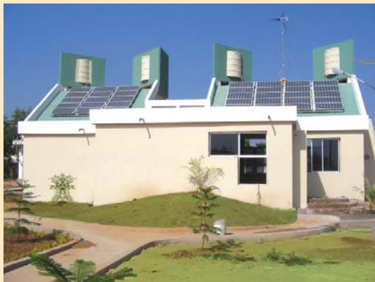
ISHBAN - the solar restaurant
